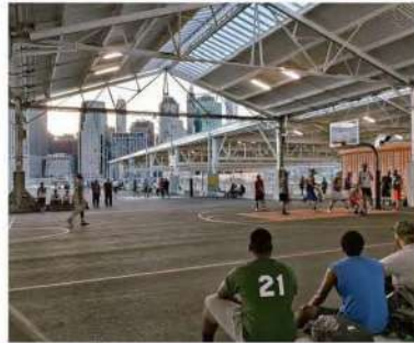
Brooklyn Bridge Park - Pier 2
