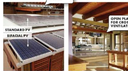
Combined cross and stack ventilation All electric solar powered building Rainwater harvested and used for bathrooms
