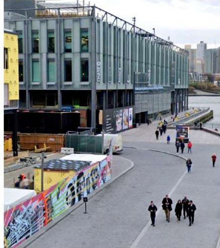
Access loop at Pier 17
