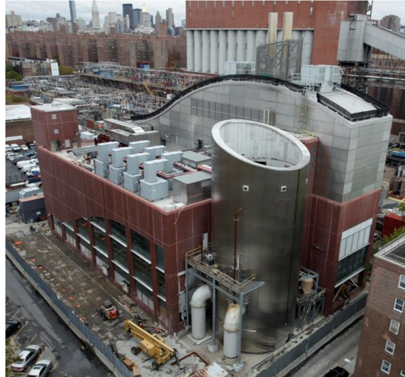
Manhattan Pump Station; Manhattan, NY Pump Station
