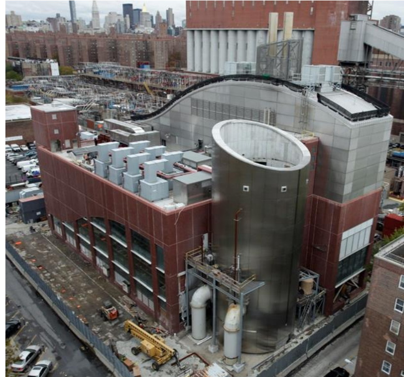
Manhattan Pump Station; Manhattan, NY Pump Station
