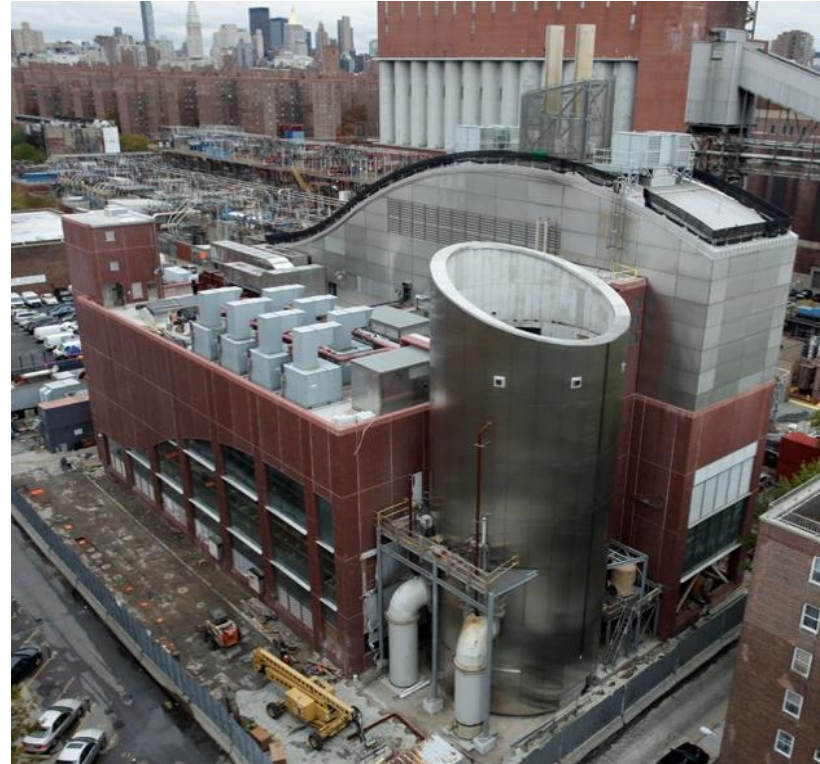
Manhattan Pump Station ; Manhattan, NY Pump Station
