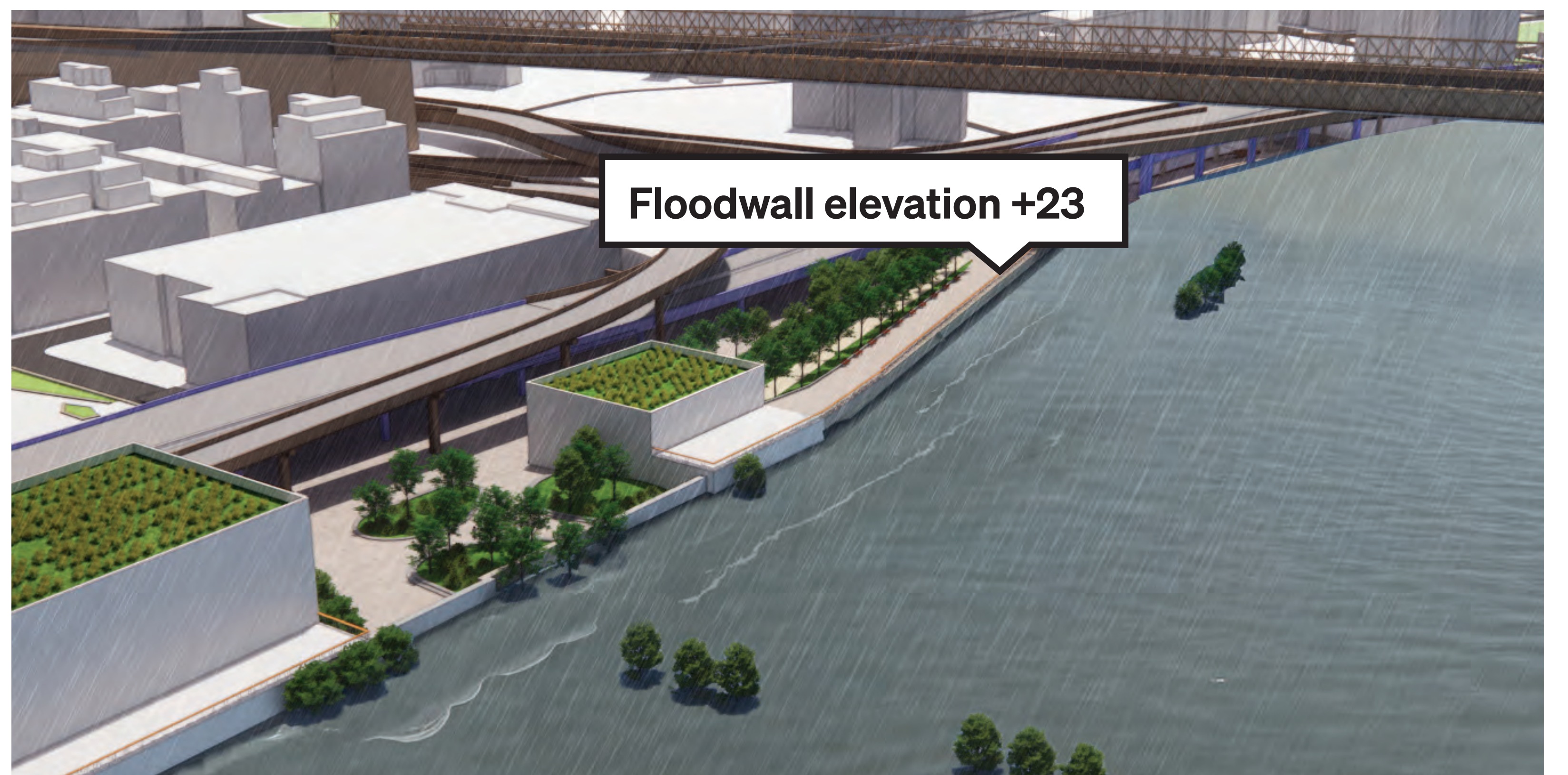
Illustration of how the floodwall and flood gates would protect Lower Manhattan during a storm.
