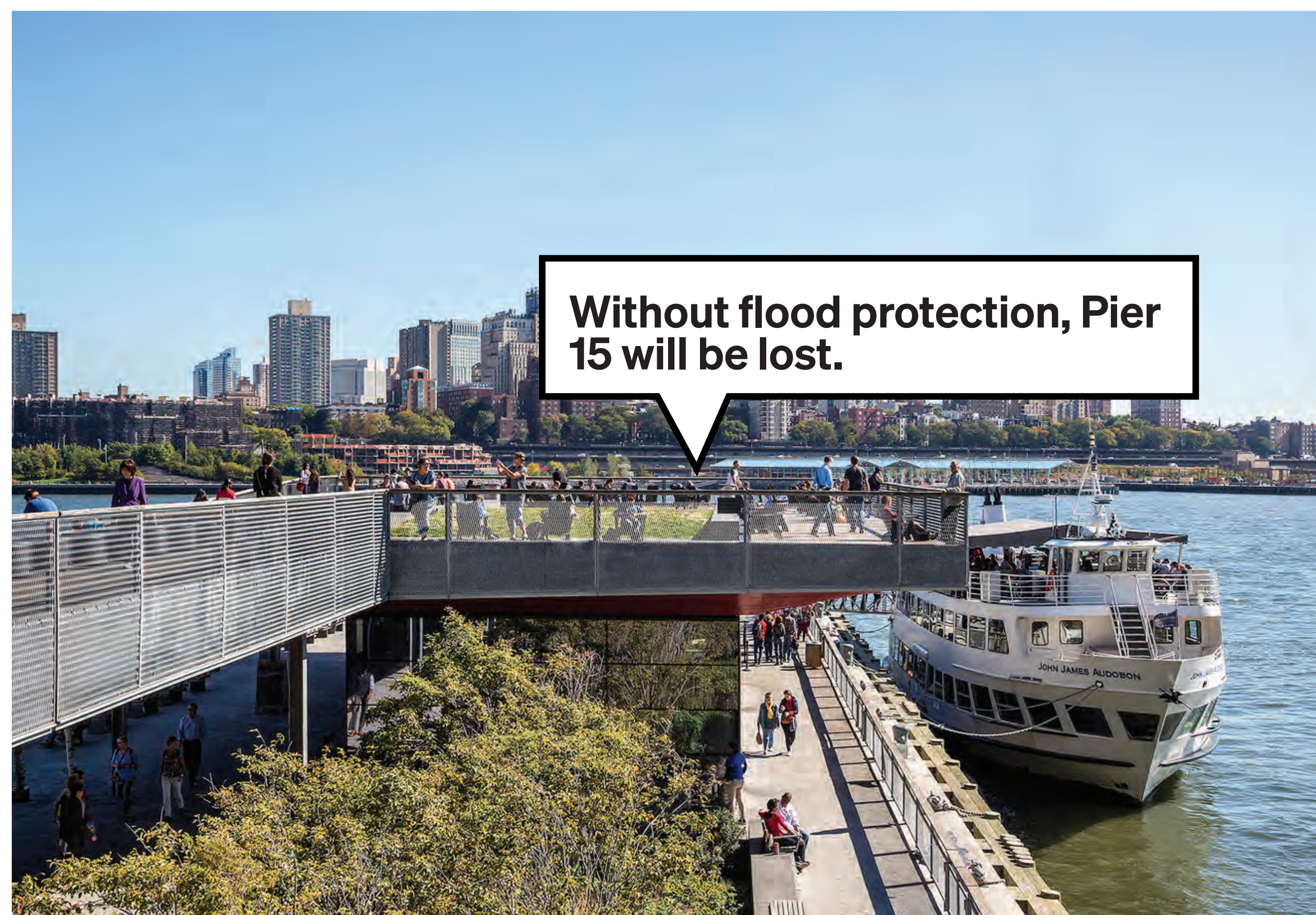
Pier 15 two-story public pier
