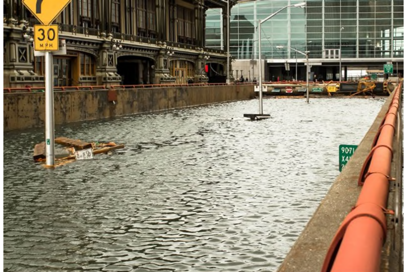
Flooded Battery Park Underpass located in study area.
